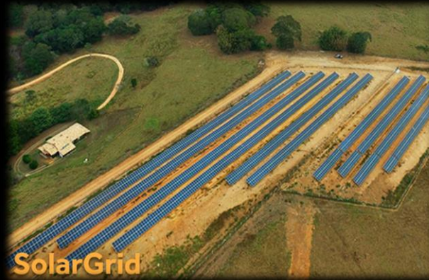
SOLAR GRID UFV - RJ
